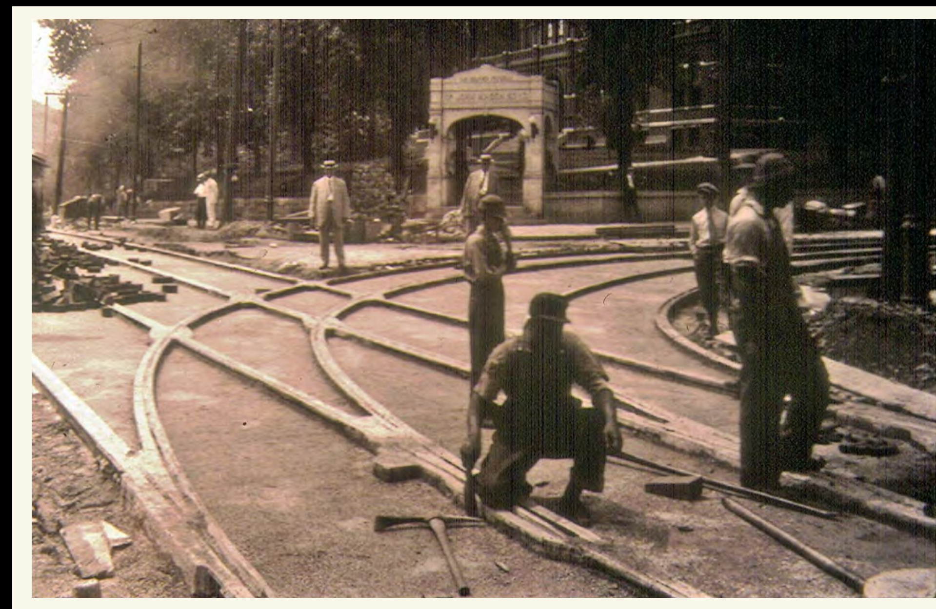
Right: Workers lay streetcar tracks at the corner of Gay St & Main St
